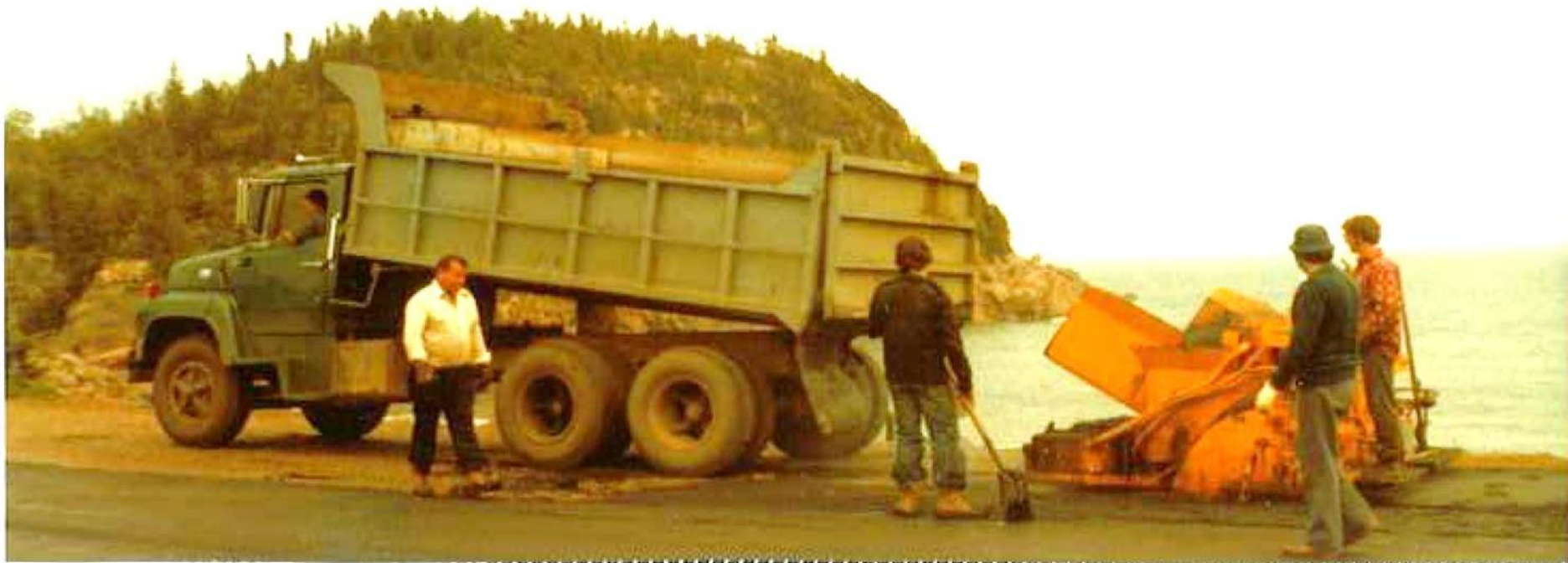
Ocean Paving at Black Brook 1977
