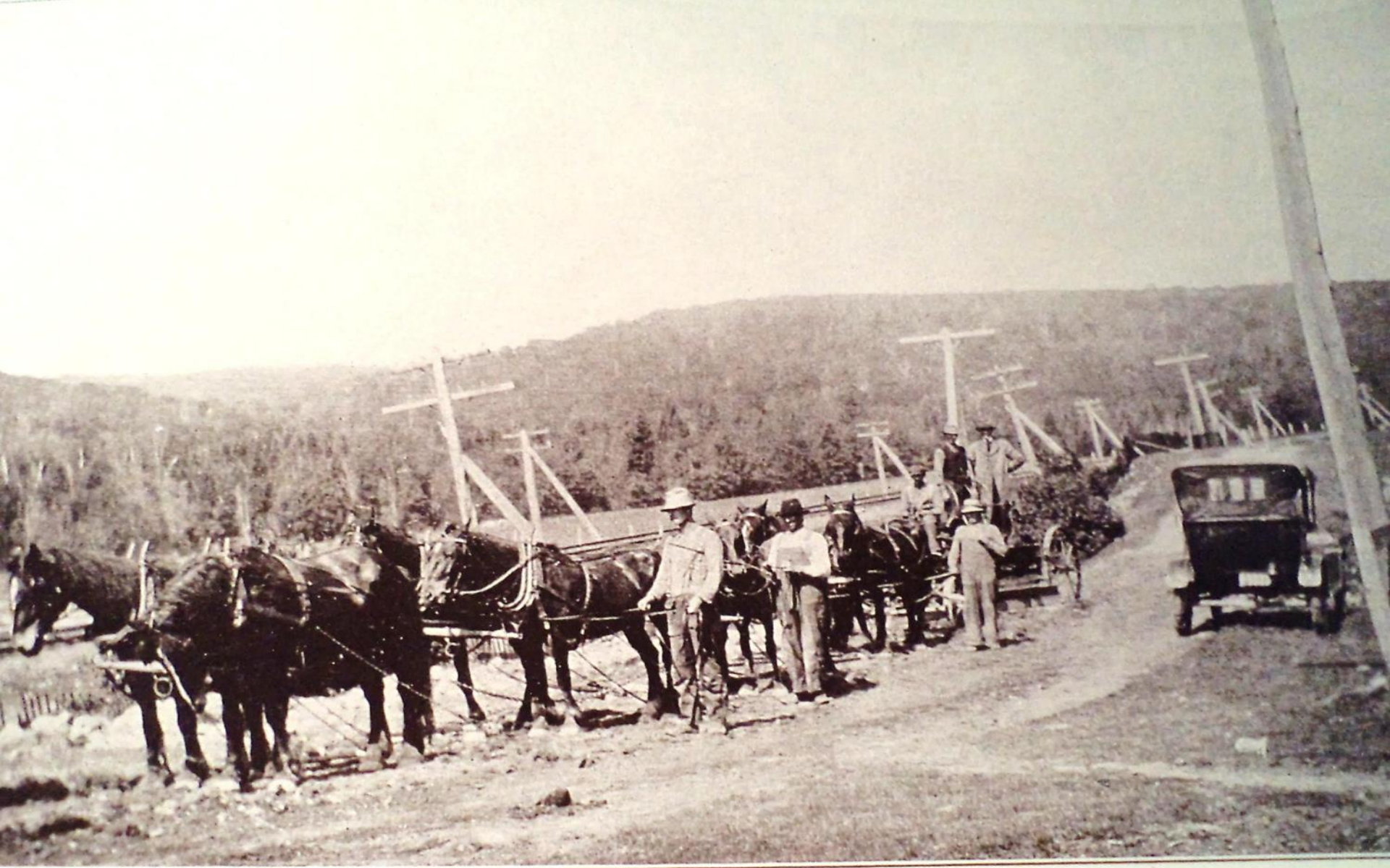
ROAD GRADER AT WORK NEAR JAMES RIVER IN ANTIGONISH COUNTY.
