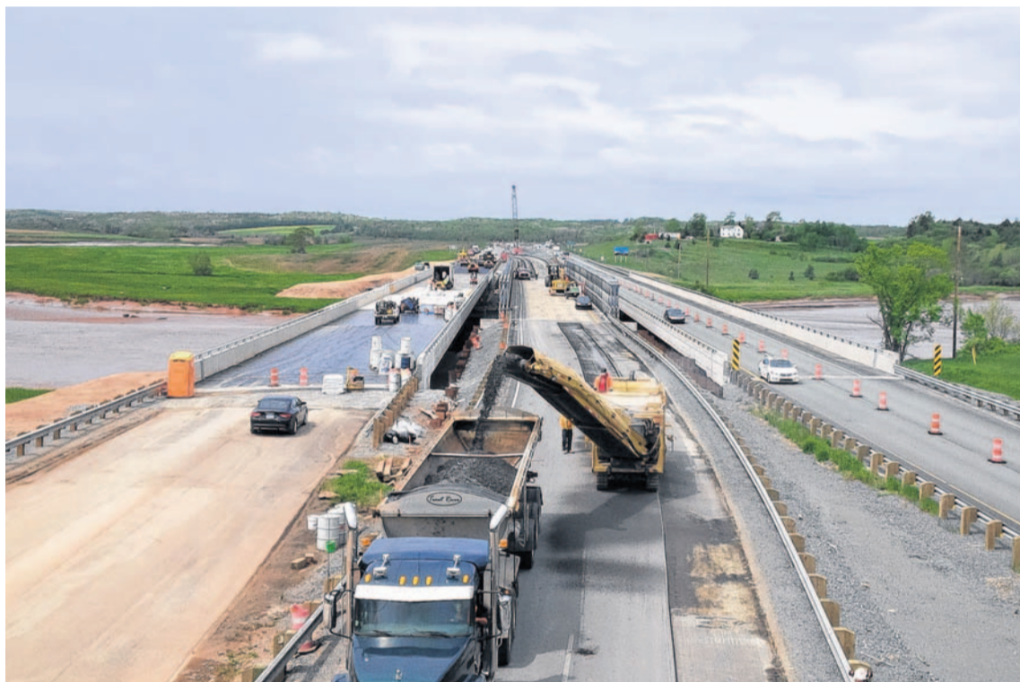
Shubenacadie River Bridge. CONTRIBUTED
