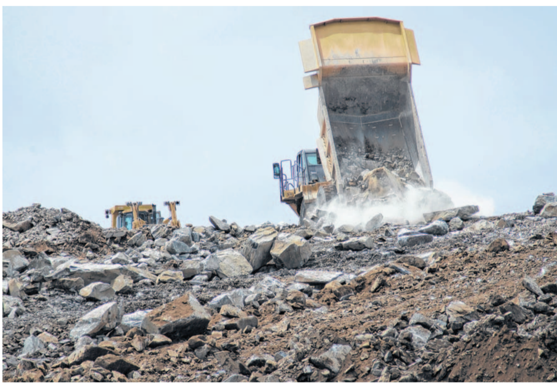
Since 2008, a collaborative program has introduced young people to the potential of jobs in all aspects of the construction industry, from labourer to CEO. CONTRIBUTED
