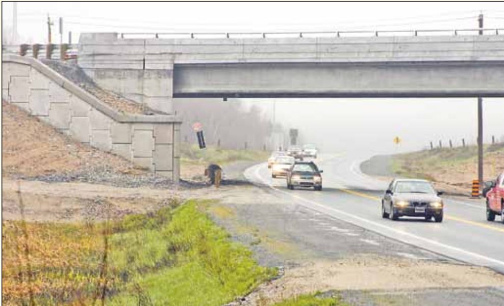
Vehicles travel under the newly constructed overpass at Exit 4 on Highway 103. Started in August, 2003, the $42-million state-of-the-art project to twin 15 km of Highway 103 from Exit 3 at Otter Lake to Exit 5 at Upper Tantallon is nearing completion.
