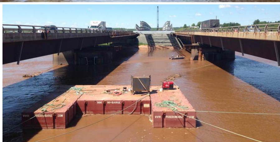
The Shubenacadie River bridges, which were built in the mid-1970s, are made out of steel girders which are in need of repair.
