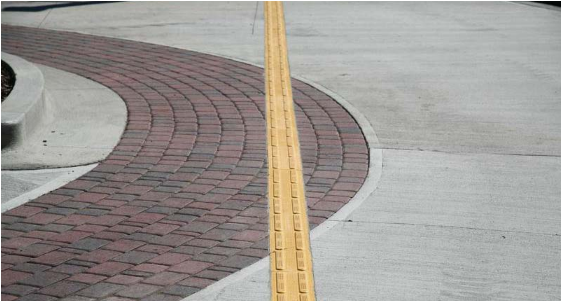
Tactile Walking Surface Indicators are typically made from metal, rubber or plastic inserts, or are built directly into concrete. Optimally TWSIs should have a texture that can be felt underfoot and detected by a long cane, and beveled edges to decrease the likelihood of tripping.
