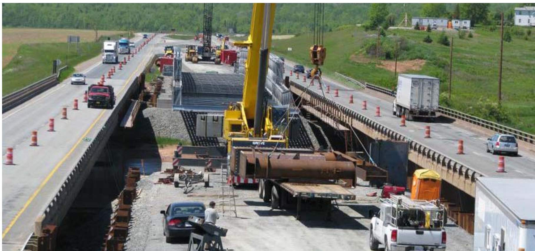
Shubenacadie River Bridge Project
