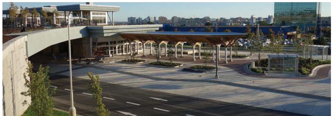
Tactile Walking Surface Indicators have been used at the corner of Alderney Drive and Portland Street in Dartmouth for a number of years, and were installed at the new Dartmouth bus terminal in 2012.
